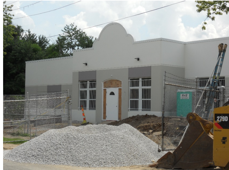
Exterior of the new building
